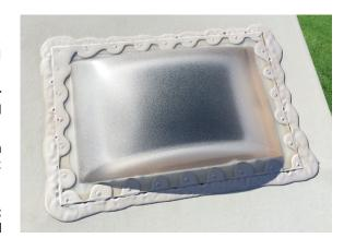
Cover all screw heads, flange and roof juncture around the entire perimeter of the skylight with an approved sealant (see caution below for additional information).
