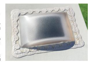
Cover all screw heads, flange and roof juncture around the entire perimeter of the skylight with an approved sealant (see caution below for additional information).
